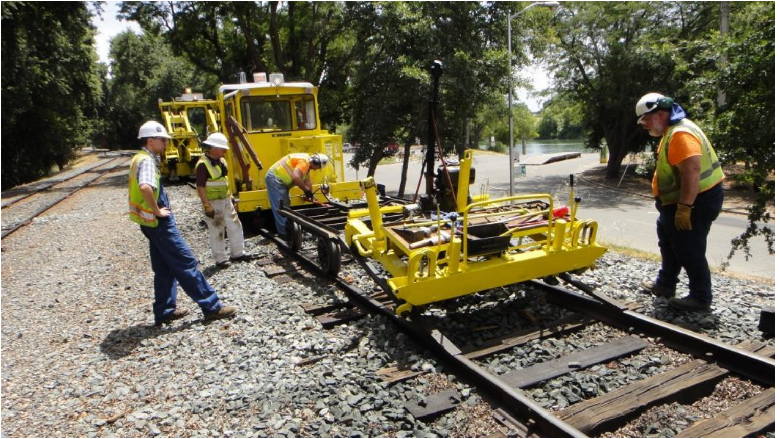
Matt, Mike H., Mike F., and Frank return the rail-lifter to its carriage
