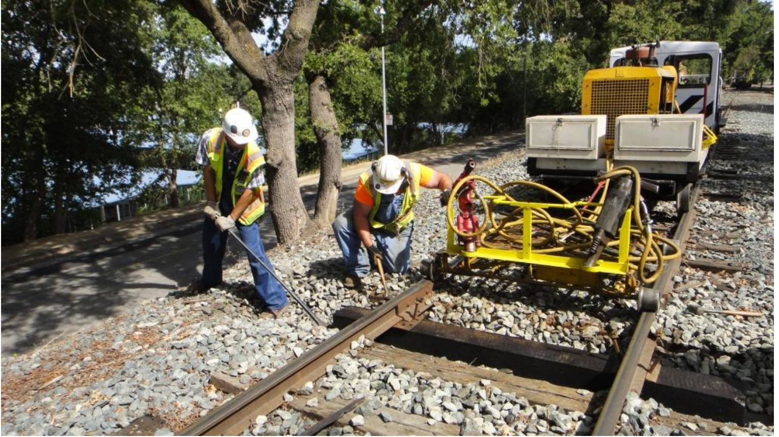
Matt nips the tie up as Mike F. resets a spike that had been out of position
