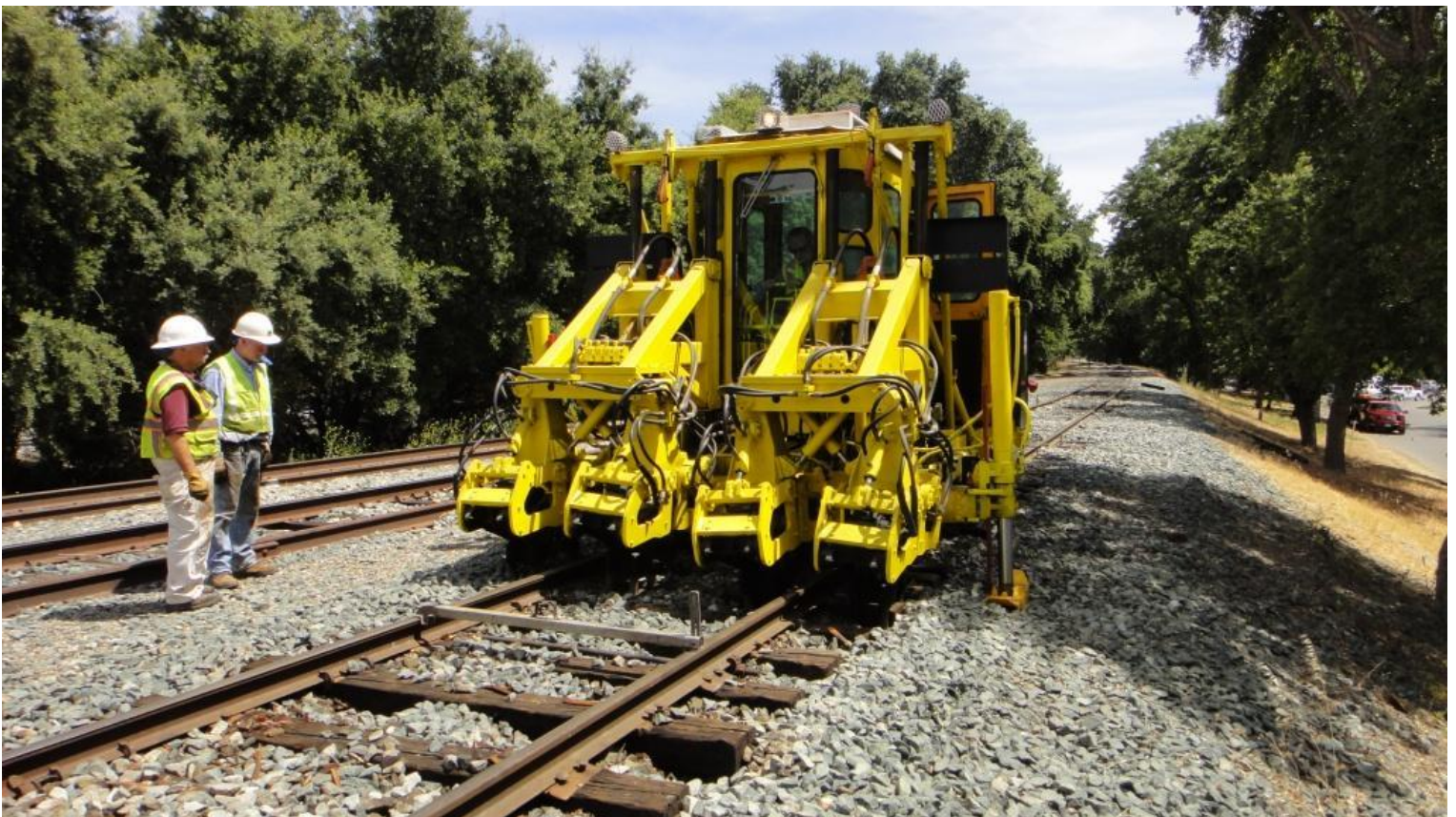
Leveling the track: the new-old tamper has a track-jacking system with which proper cross-level can be achieved
