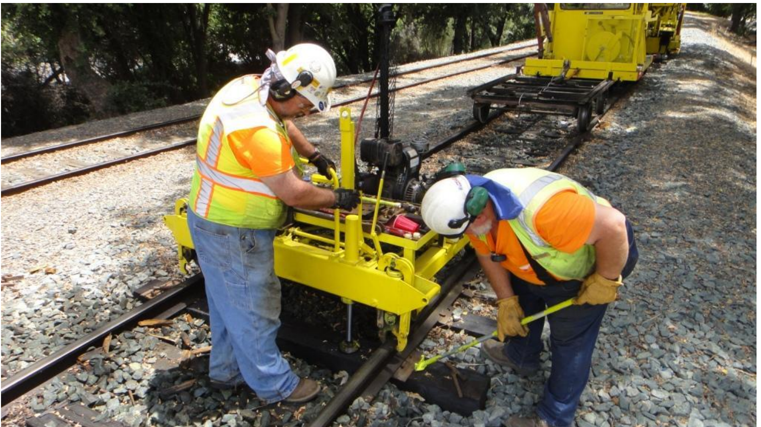
Mike F. and Frank use the rail-lifter to insert tie-plates
