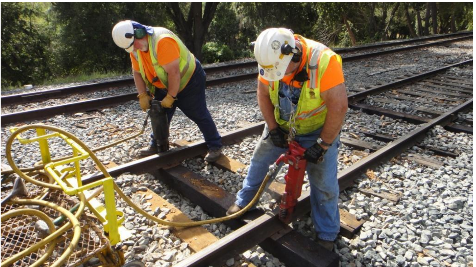
Synchronized-spiking: Frank and Mike F. take the first spiking shift. Those things weigh 60 pounds each – plus hoses...
