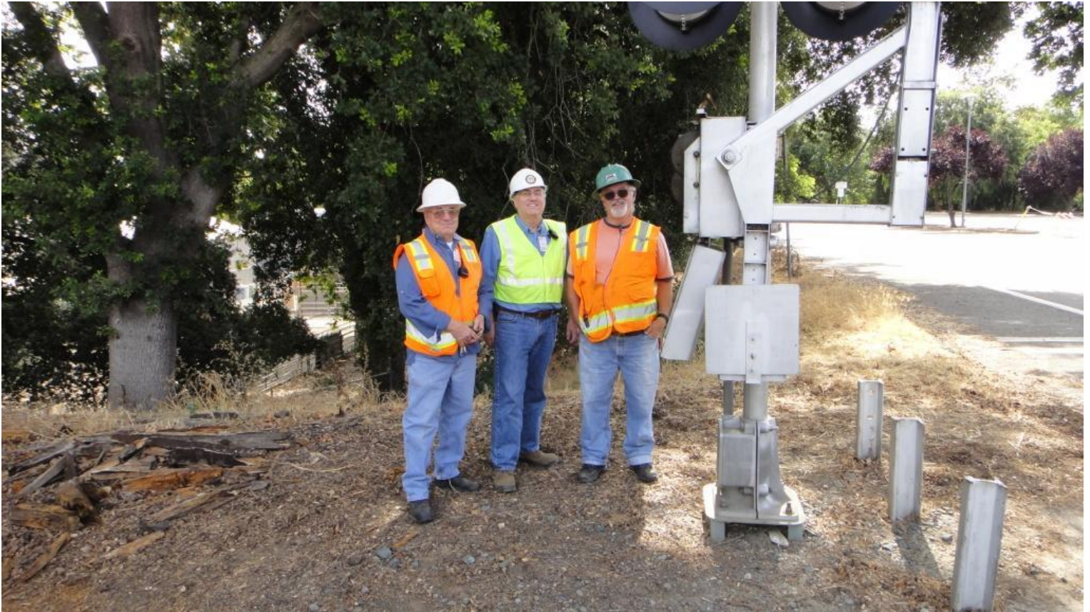
Signal Department's, Joe Galipeau, Mike Gaulke, and Al Utzig manned the Front Street grade-crossing warning system
